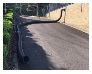
Commission decided to study the problems, again. It was noticed that at least part of the rainfall collected by the roof over that section of the church building runs out of a spillway and runs down the side of the building and onto the curb/pavement. That spillway correlates generally with the areas inside suffering moisture problems. It was also noticed that the moisture problems along the ground side wall of the hallway running past the rector's office also correlates with the spillway.
