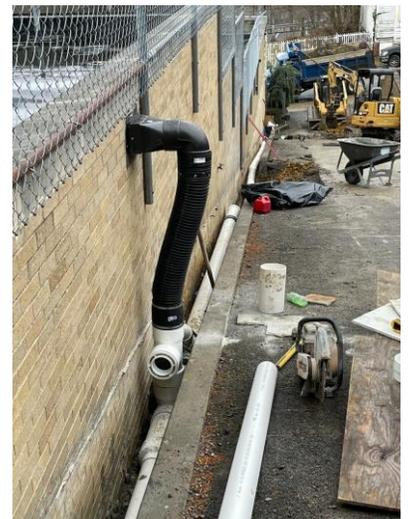
then run a new PVC drain pipe down the exterior wall and tie it into the storm drain. Then a French drain was installed above the drain pipe and the concrete curbing between the wall and driveway was reinstalled.
